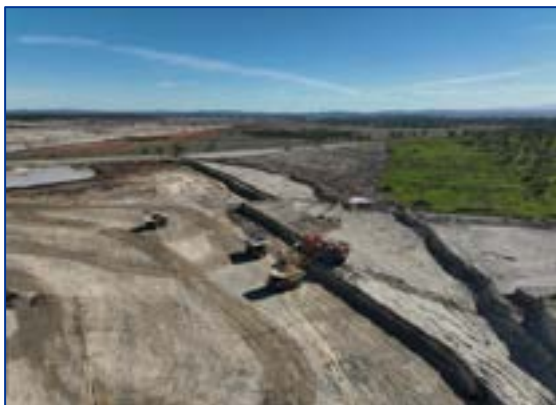
Plate 1-3 – Initial Excavation of Box Cut
